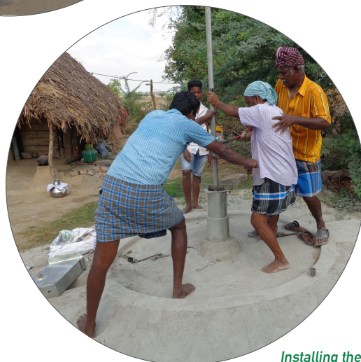
Installing the hand pump
